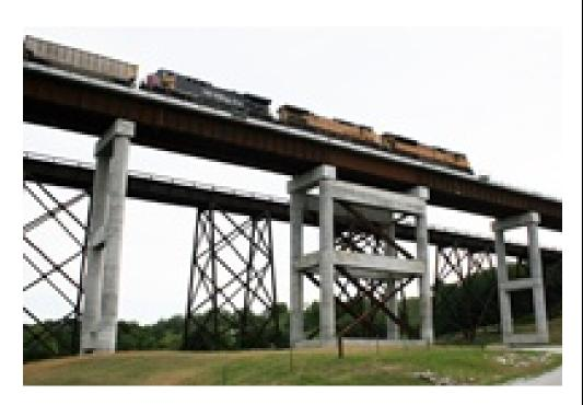
The bridge carries trains of UP's "Central Corridor," which links Chicago with the West Coast and the Powder River Basin coal fields. Trains crossing the 1901-built Kate Shelley bridge had to slow to 25 mph, making it a bottleneck on the busy line. When completed, the new bridge will be able to handle 70 mph trains.
