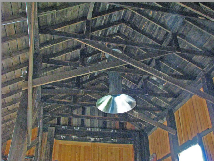
interior photos for structure reference
